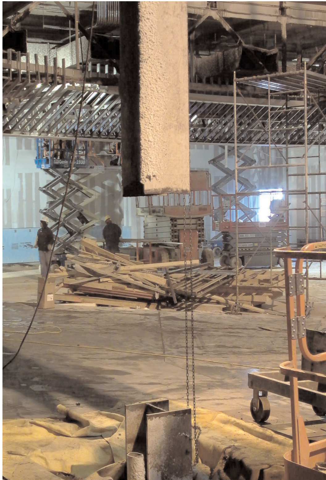
Right: The cut column no longer helps support the structure and now the load of the FBA Worship Center is securely resting on the new engineered foundation support system.
