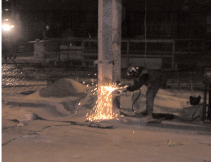
Above: Torching one of the central support columns to open the view inside FBA Worship Center.
