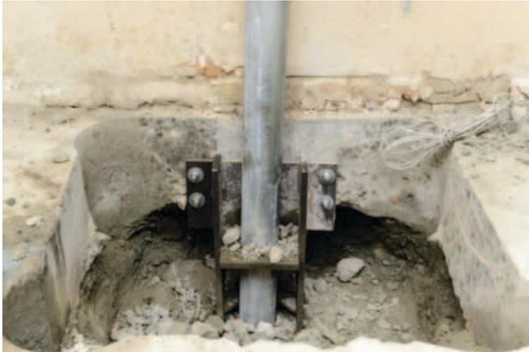
lead section of the pier reduces skin friction on the pier pipe during installation. The pier capacity is primarily from end bearing on a hard/dense soil stratum. The ATLAS RESISTANCE® Pier has been successfully driven to depths of 200 feet to ensure proper and verified support.
