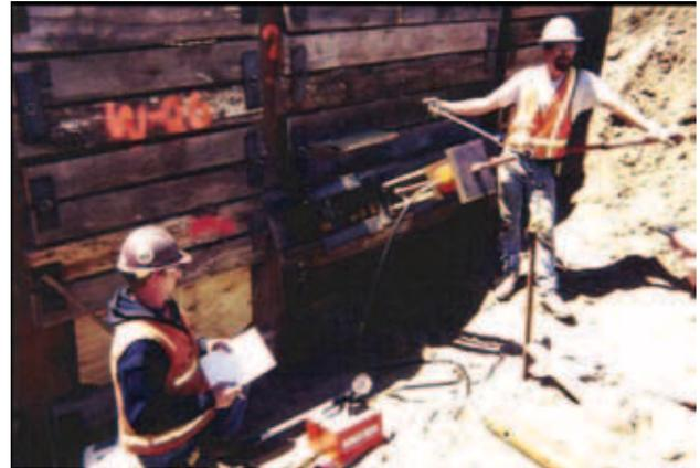
Anchor Tension Load Test in Minneapolis, MN
