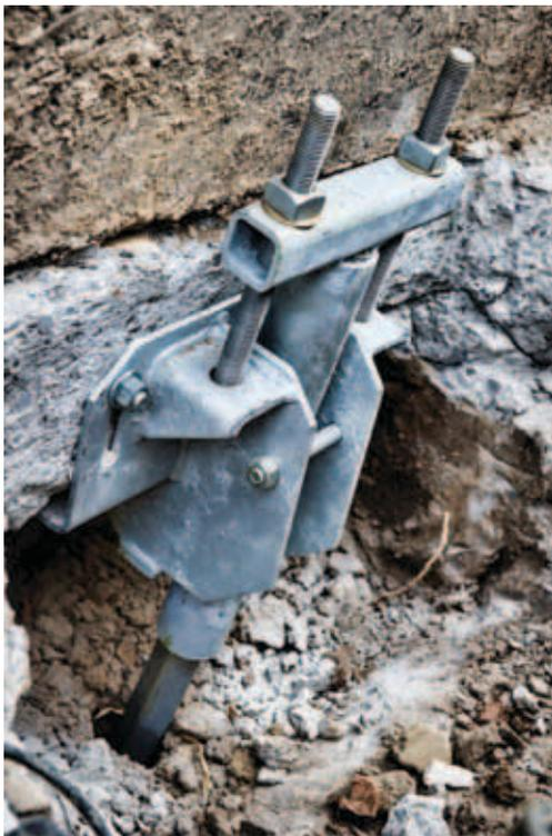
More recent developments include the SQUARE ONE® (1980) and the TOUGH ONE® (1989) patented guy anchor families with 10,000 and 15,000 ft-lb installing torque capacities. Unlike previous PISA® designs, these anchor designs are driven by a wrench that engages inside, rather than over, their welded socket hubs. Both use the PISA® extension rods with threaded couplings.
