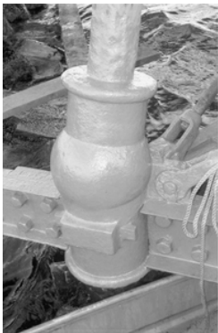
Cast iron coupling at Thomas Point Lighthouse
