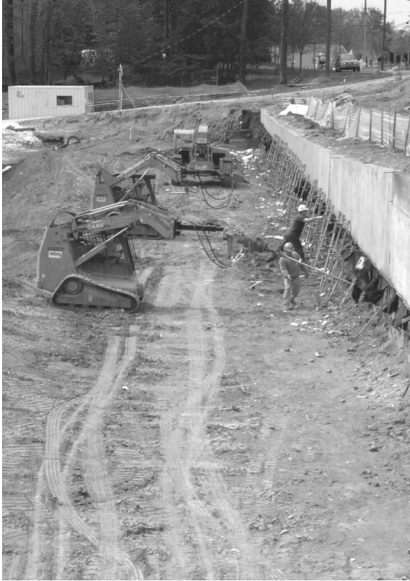
Two skid steer machines are shown above installing a second row of ECP Soil Nails.
