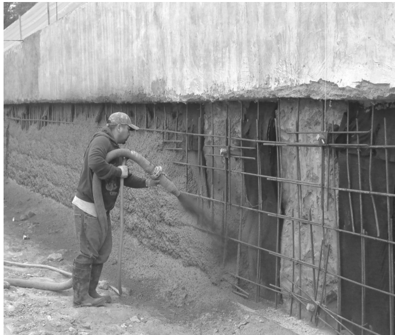
The photographs show ECP Soil Nail installation and Shotcrete application.
