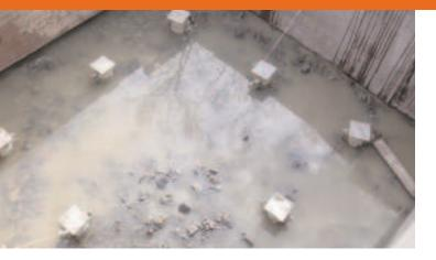
■ The depth of suitable bearing strata was estimated at approximately 50 feet below the proposed top of the pier elevation. Galvanized materials were recommended based on the soil conditions of the site.
