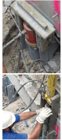
each pier and recorded on the field log. The actual verified Factor of Safety between installation pre-load and final lock off can then be confirmed. Table 6-1 is an example of the driving (installation) and lift forces that could be involved in the installation of ATLAS RESISTANCE<sup>®</sup> Piers.
